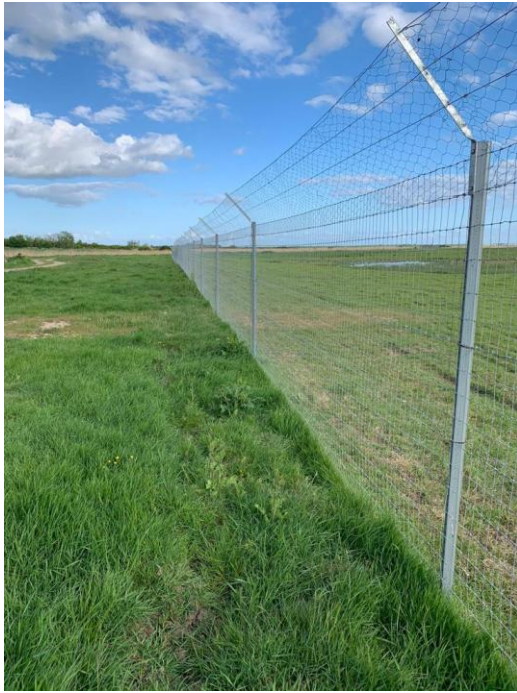
Figure 3-1. Example of a fox proof fence installation. Note that the vegetation along the outside edge (left hand side of the photo) has fully recovered following replacement over the buried skirt.
